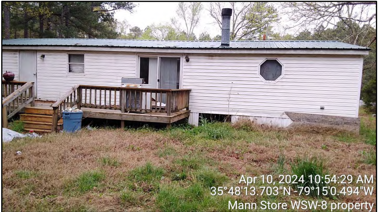
View of the rear of the WSW-8 residence, facing west.
