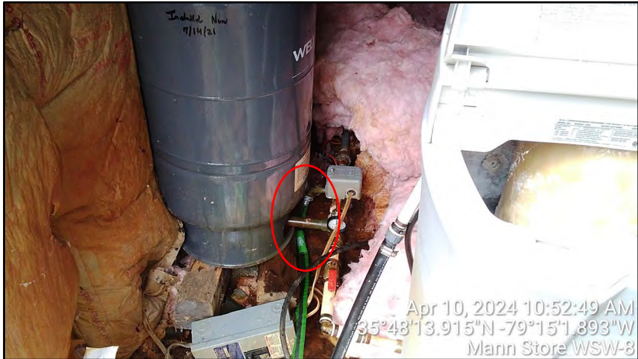
View of WSW-8 sample point. (Spigot is where green hose is connected in the photo.)
