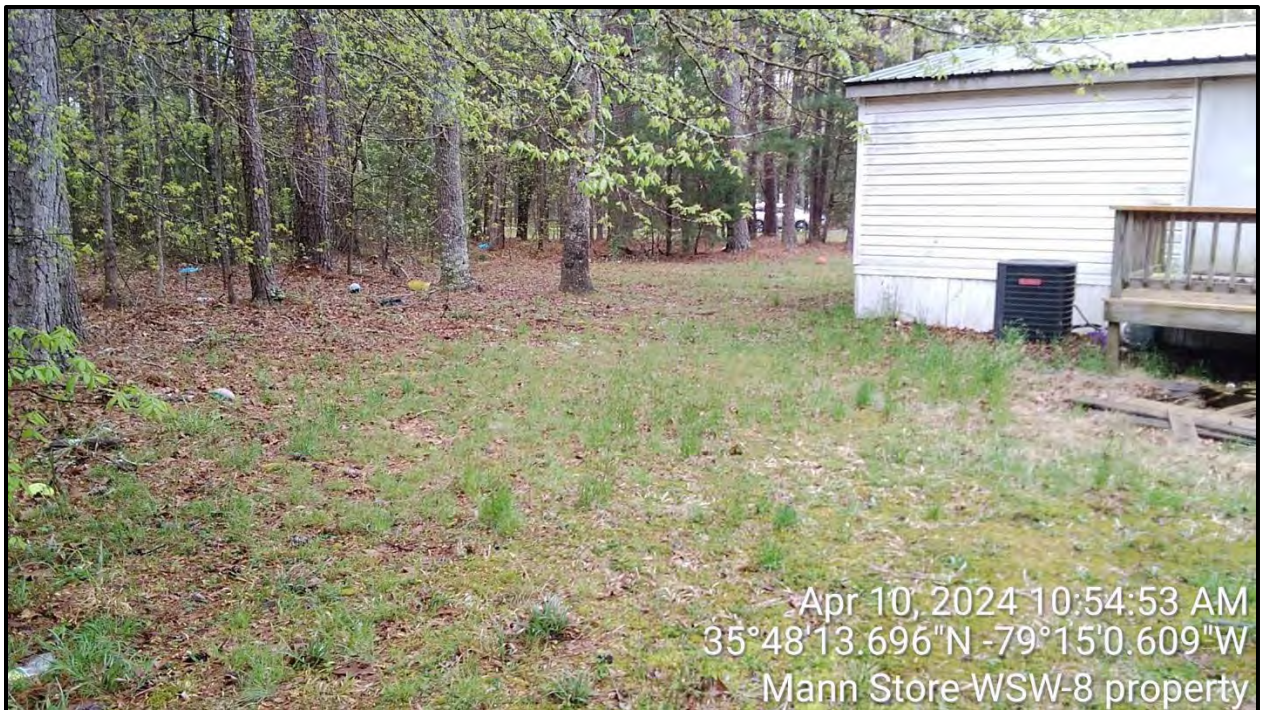
View of the rear of the WSW-8 residence, facing southwest.
