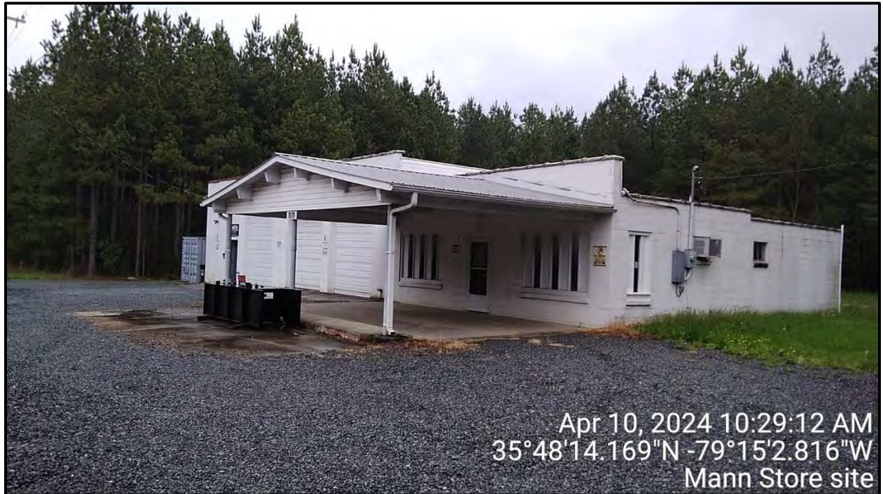
View of site, facing northeast.
