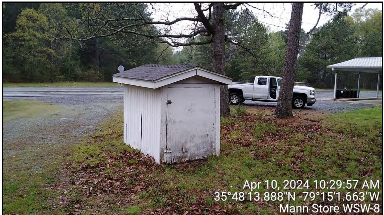
View of WSW-8 well house, facing northwest toward NC 87.
