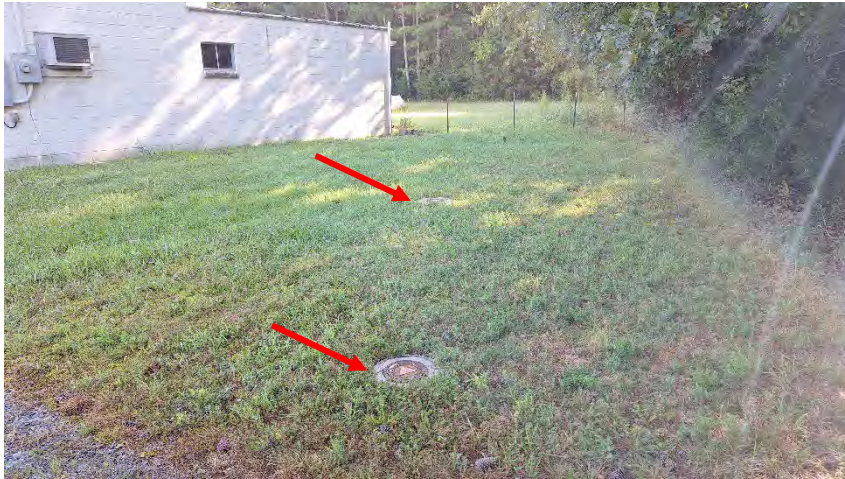
#13 – Additional Monitoring Wells, South of Mann Store Site
