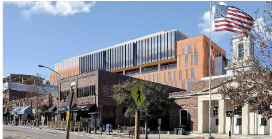
Grubb Properties + Perkins Eastman - East Roesmary St. Office & Research Bldg.
