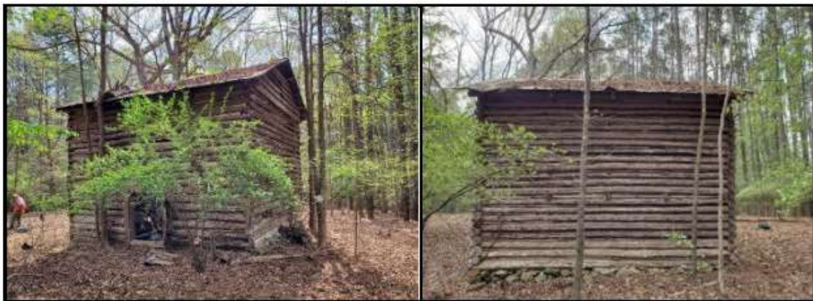
Figure 28 | Barn 1 and Barn 2 at Site 31CH1367
