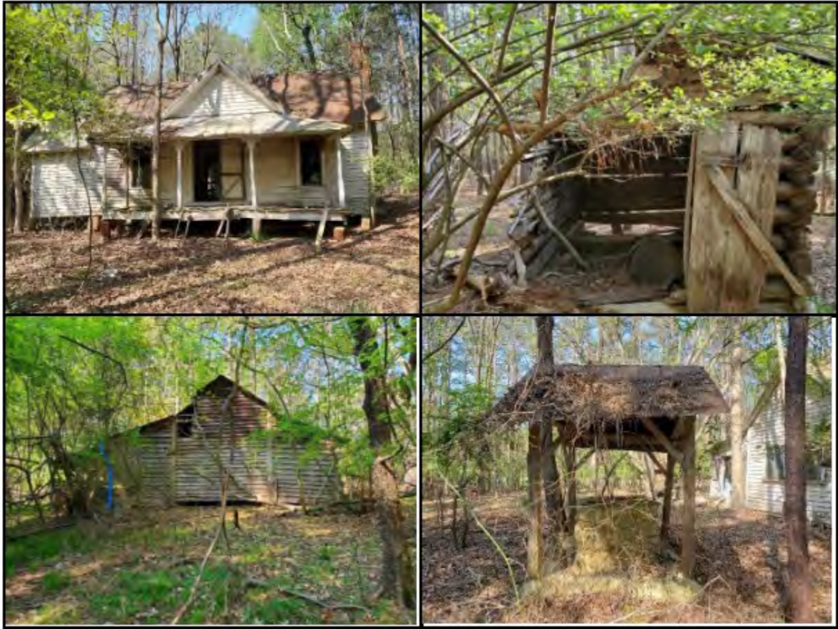
Figure 29 | Buildings at Site 31CH1366 (Top: Building 1, Building 2. Bottom: Building 4, Building 3)
