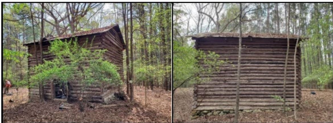
Figure 28 | Barn 1 and Barn 2 at Site 31CH1367
