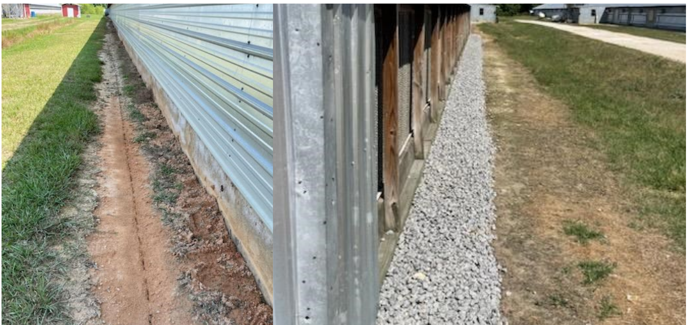
Rooftop Runoff Management Before (left) and After (right).
