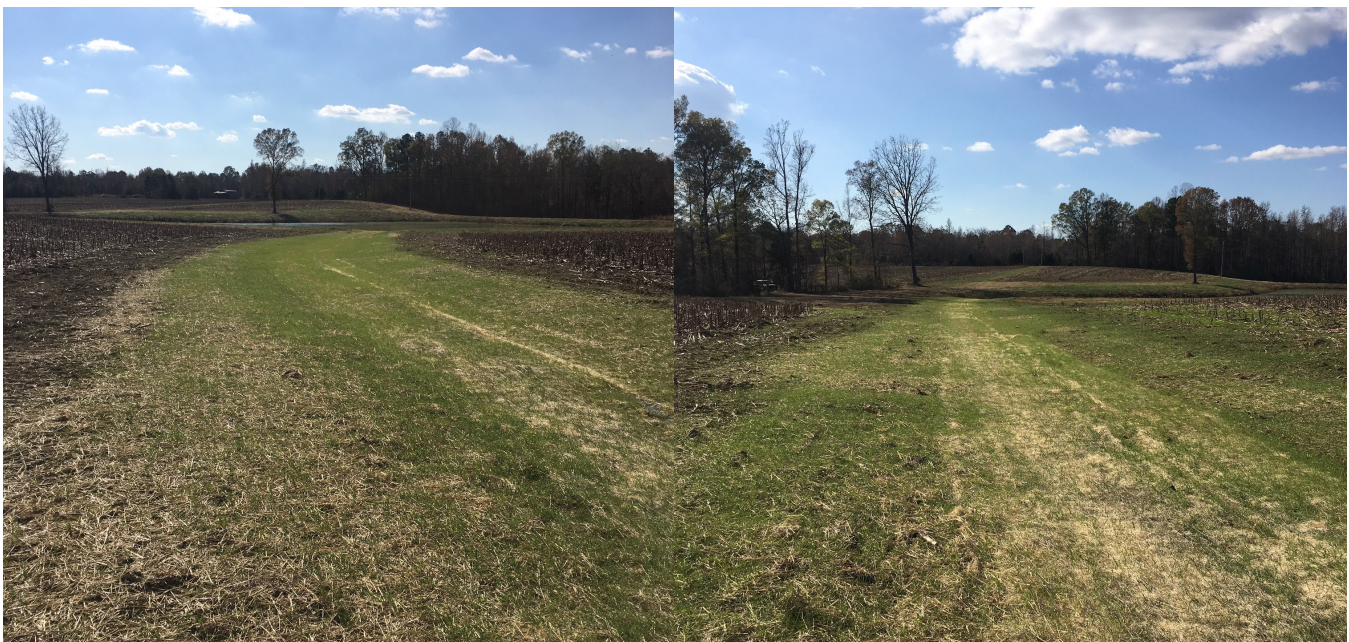
Completed Grassed Waterway
