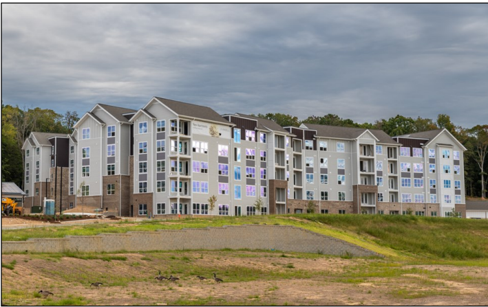
The Knoll Apartments, US 15-501 and Taylor Road
