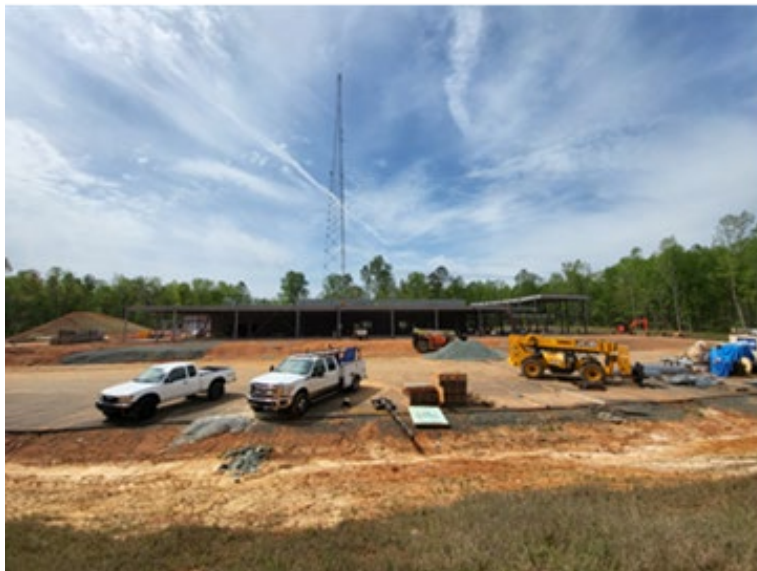
New Emergency Operations Center (under construction!)
