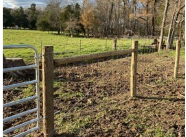
Completed Livestock Exclusion Fencing
