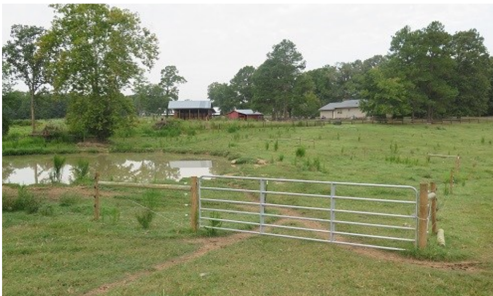
Completed Livestock Exclusion Fencing
