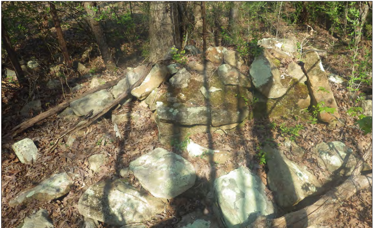
B. The Intact Portion of Chimney Fall in the Rubble (Facing North)
