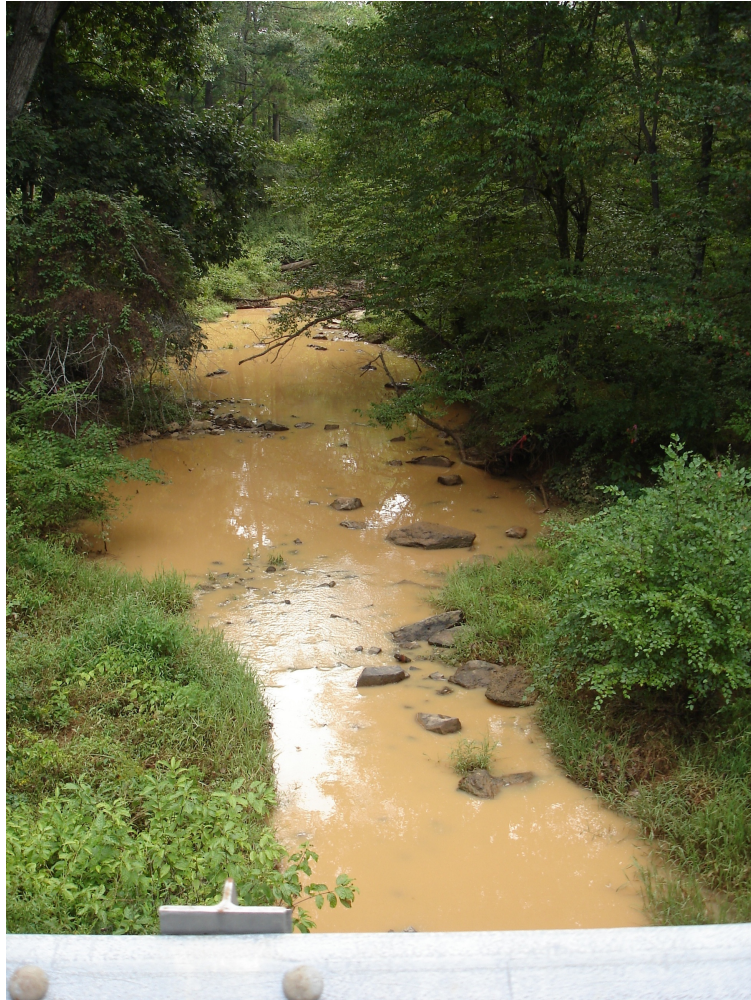
Muddy waters flow under Old Graham Road bridge at Dry Creek September 7, 2006. Photo by Elaine Chiosso
