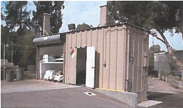
An example of a fertilizer and pesticide storage facility.
