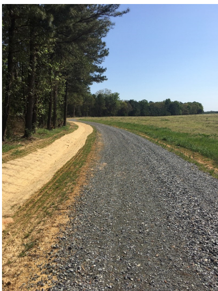
Completed Critical Area Planting
