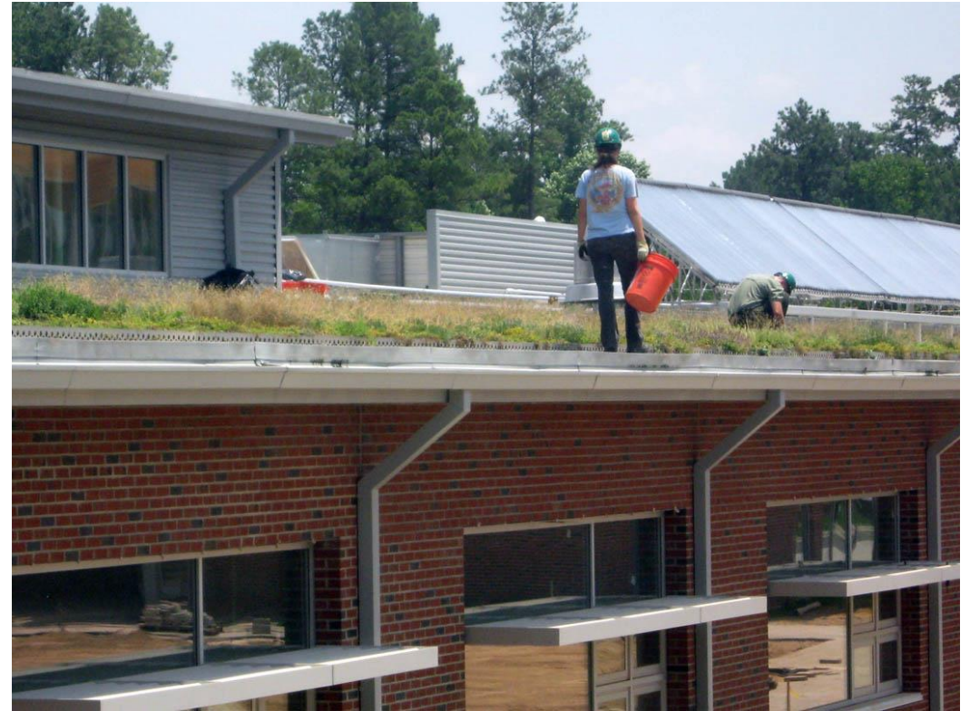
Solar water heater and vegetated roof at the CCCC Sustainable Technologies Center
