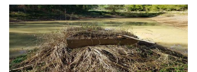
**11/2/19** Corrective actions needed, work can only proceed if baffles are installed in the sediment basin and ditch within 7 days
