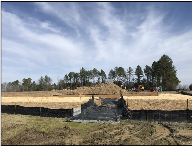
Expansion of Floorazzo, Siler City
