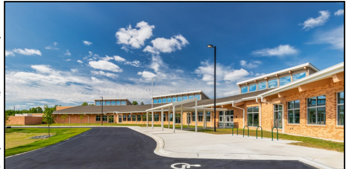
Chatham Grove Elementary School, Pittsboro
