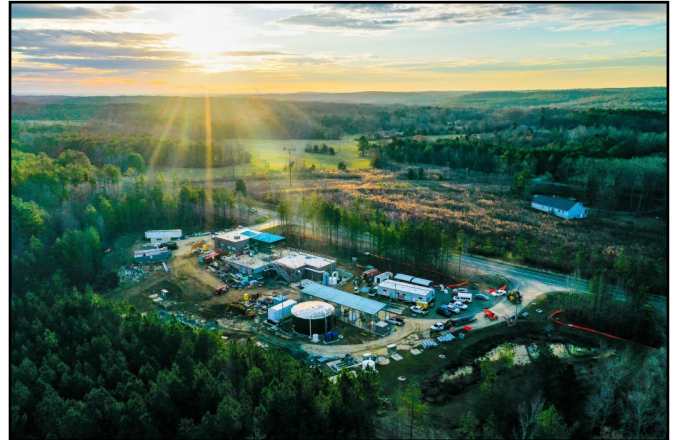
Chatham Park is a 7,100 acre planned mixed-use development located adjacent to Jordan Lake and Pittsboro. At full build out, the project is expected to add 60,000 residents and to house 22 million square feet of office, research, retail and community space.
