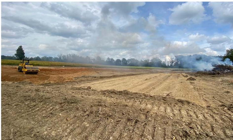
Irrigation Pond Construction in Progress
