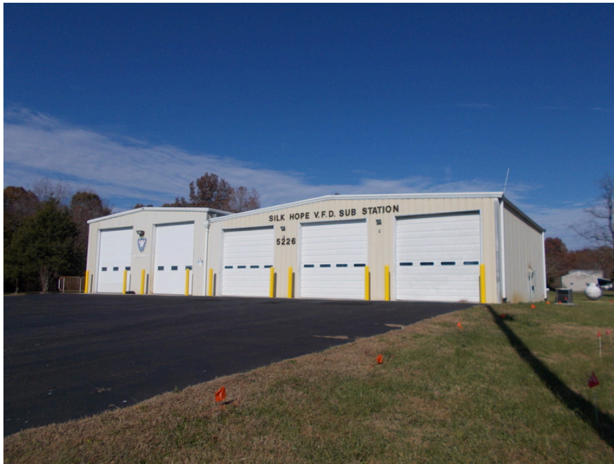
Site Photograph 17 – Fire Department
