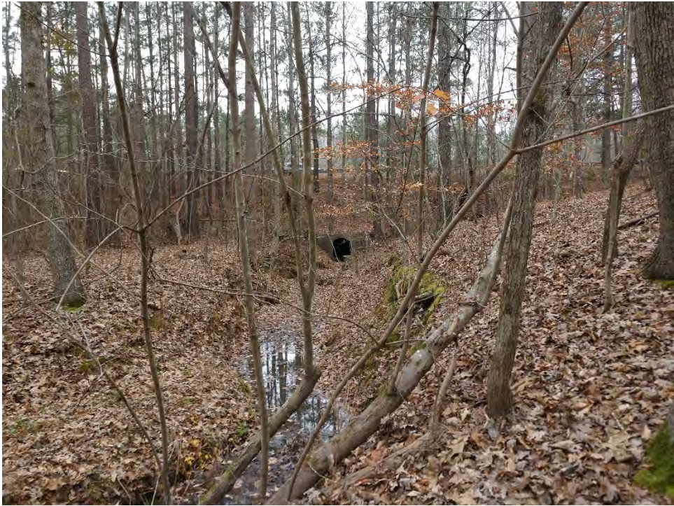
Photo 1: View of Stream A as it enters the US-1 culvert.
