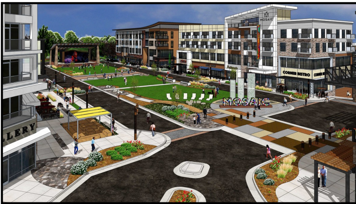
The MOSAIC is underway in Pittsboro. The development is expected to be the epicenter of Chatham Park.
