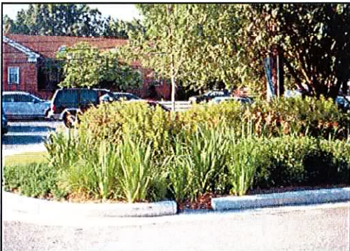
Bioretention areas in parking lots can help retain stormwater runoff on site and filter out water-borne pollutants.
