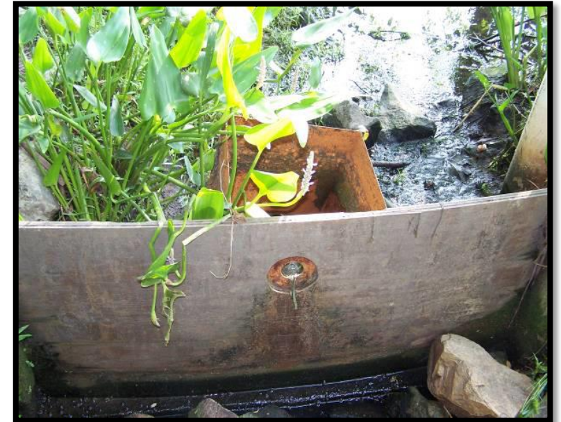
Flashboard Riser Outlet One wall of riser have movable boards to adjust water levels
