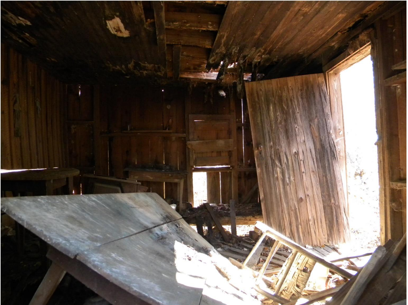
Interior of shed addition.
