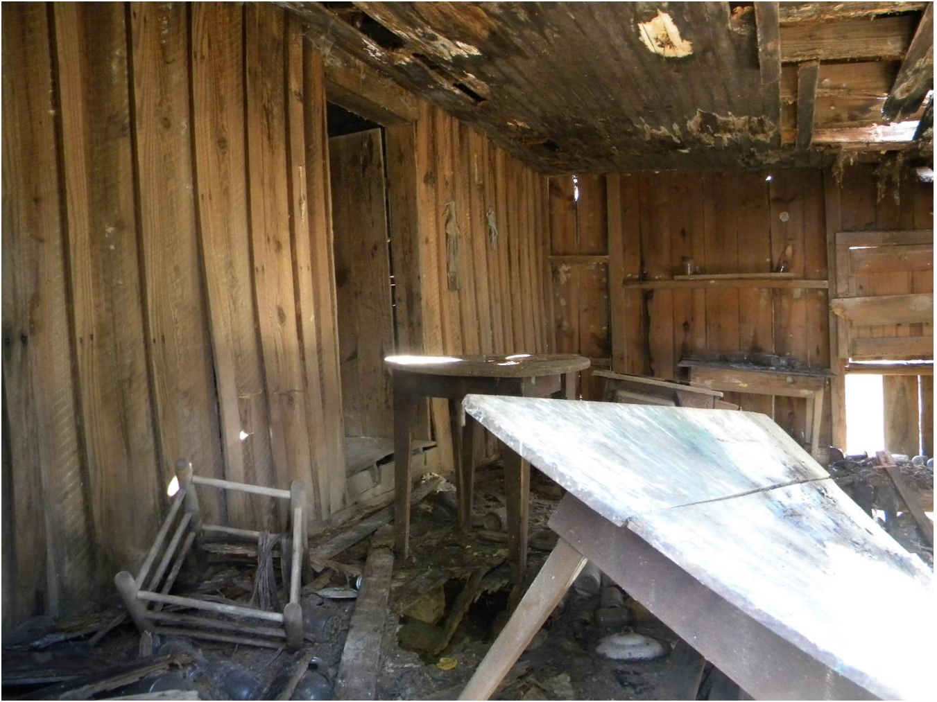
Interior of shed addition.
