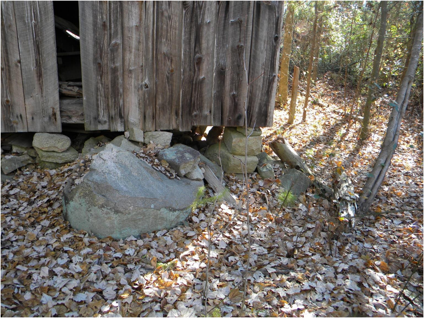
Shed addition. Looks like they built to accommodate the large boulder.
