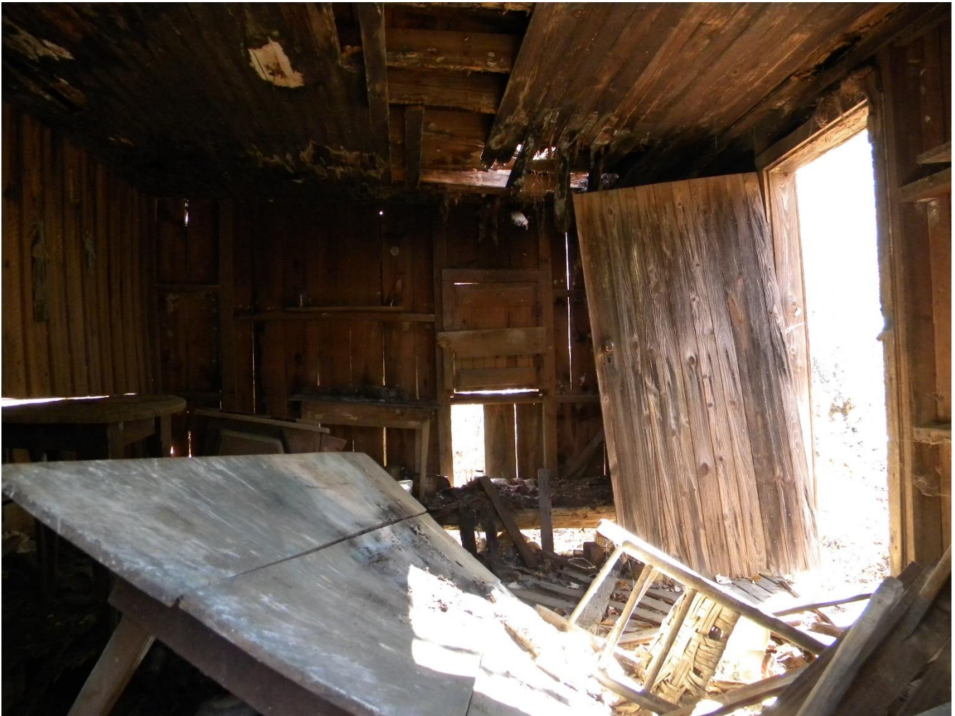
Interior of shed addition.
