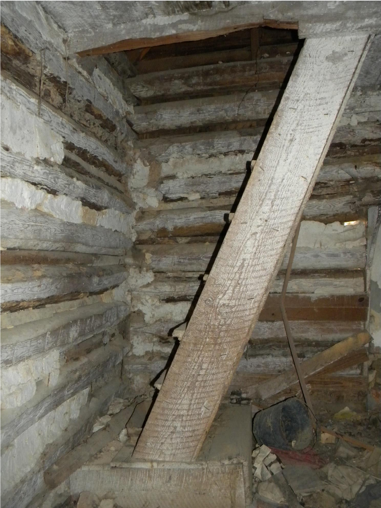
Stairs to loft
