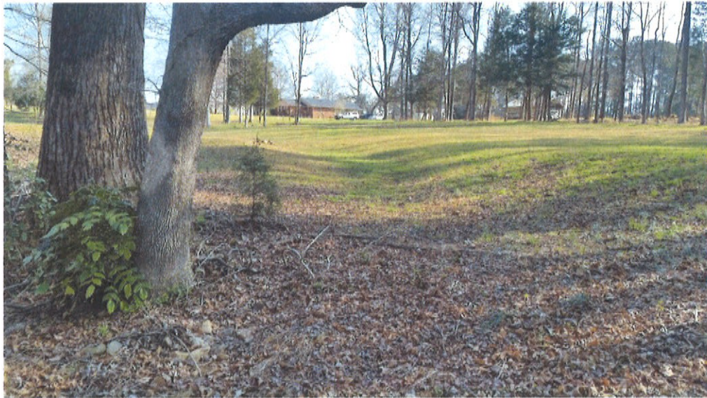
Photo 5: Emergency spillway. Up gradient view.
