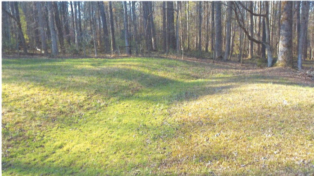
Photo 4: Emergency spillway. Down gradient view.
