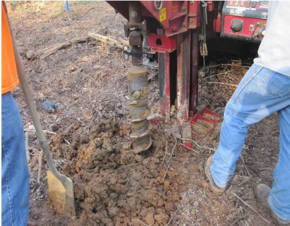
5. Creation of Borehole
