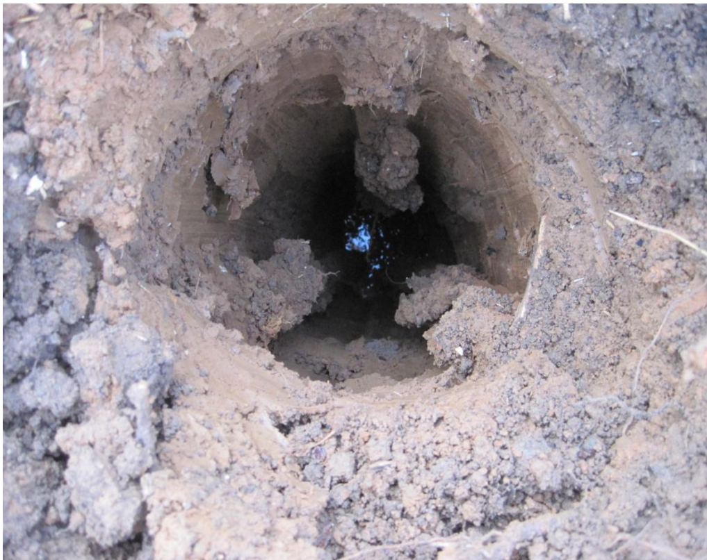
6. Creation of Borehole #2
