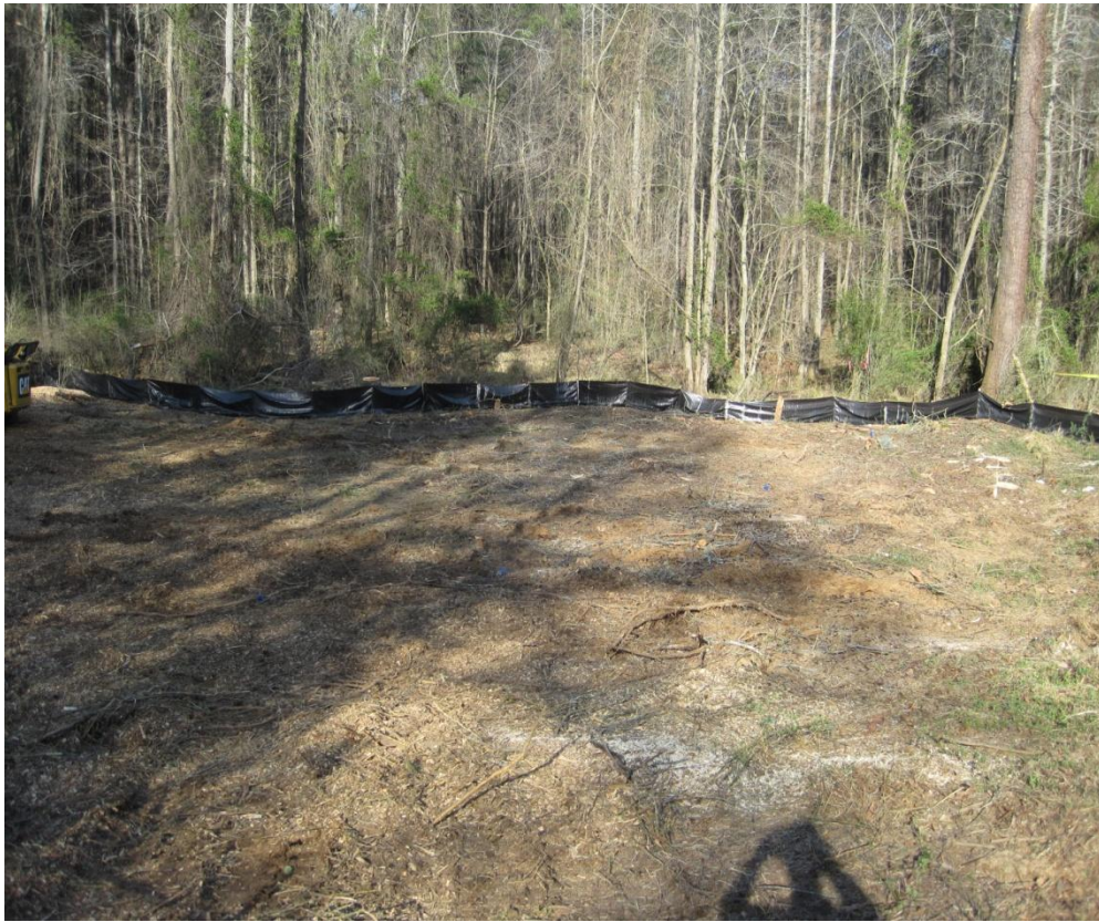
3. Sediment and Erosion Control: Silt Fencing
