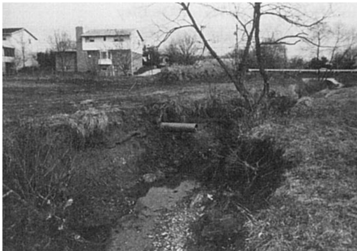
Streambank Erosion Fills Streams With Sediment.
