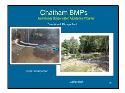
On the left is a photo of the diversion, which created a stable drainage way for the water that leads to a plunge pool. The large rocks in the plunge pool serve as a means to slow down the velocity of the water, which decreases its erosiveness. On the right is a current photo taken this spring. Here we are standing at the foot of the plunge pool looking up into the diversion.
