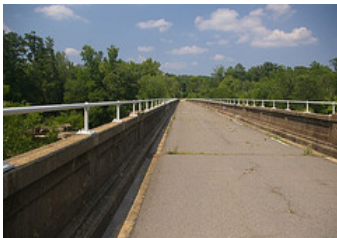
Figure 8: Old Bynum Bridge
