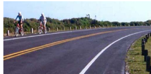
Figure 40: Example of a wide paved shoulder
