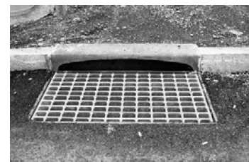
Figure 46: Bike friendly drainage grate
