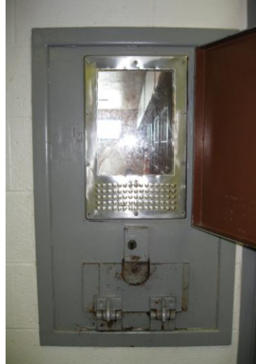
The outer undersized window and a smaller one on the door are the only visual viewpoints into the cellblock.
