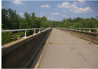
Figure 7: Old Bynum Bridge
