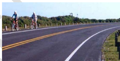
Figure 35: Example of wide paved shoulder
