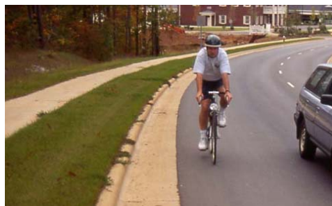
Figure 36: Example of wide outside lane
