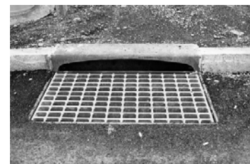
Figure 44: Bike friendly drainage grate
