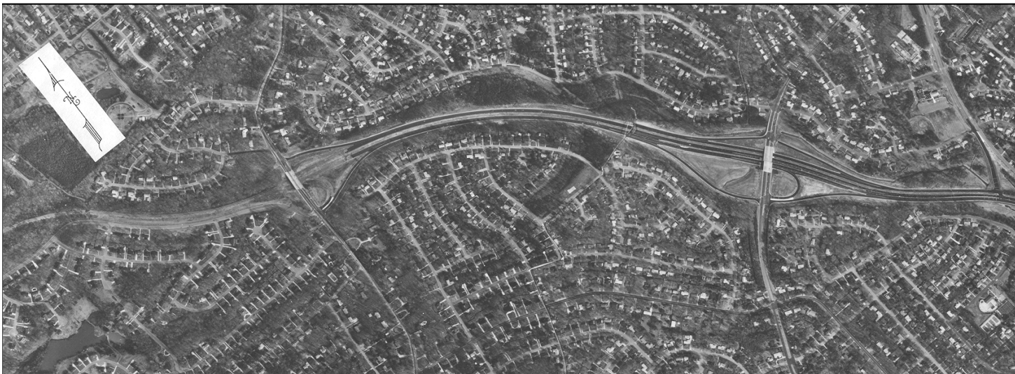
Benjamin Parkway after construction in 1990
